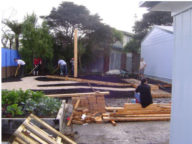
SOME OF THE GARDEN BUILT BY THE ANZ BANK VOLUNTEERS
